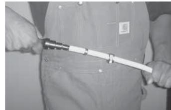
4. Push the fitting onto the pipe and fully against the shoulder of the fitting. If necessary, at this point the fitting can be rotated on the pipe to facilitate threading onto a valve, tee, etc.
