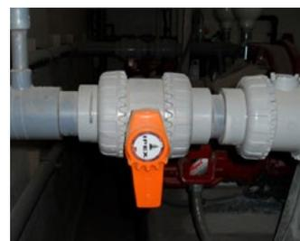
IPEX manual VXE, VX and electric actuated VKD Series Ball Valves were used throughout the facility to control flow as needed.
