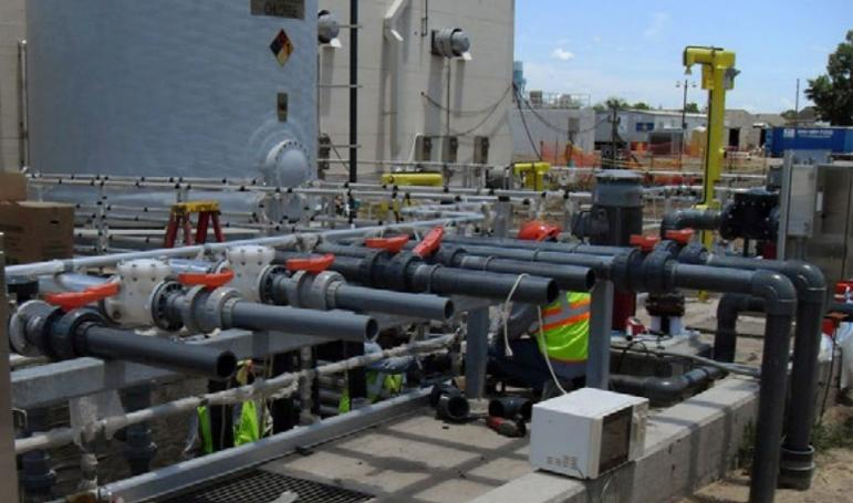
IPEX Corzan® CPVC pipe, valves and fittings are used in areas transporting highly-corrosive chemicals.
