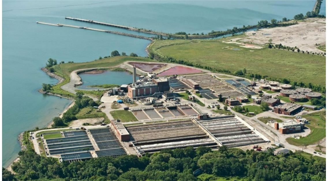
Originally built in the late 1950s to handle an average flow of 2 million gallons per day (mgd), the G.E. Booth (Lakeview) Wastewater Treatment Plant (WWTP) is a key facility for the Region of Peel. In 2009, the facility underwent a \$260 million expansion to treat 137 mgd from the more than 1.3 million residents and 90,000 commercial businesses in the eastern section of Mississauga, Brampton, Bolton, and Caledon East.
