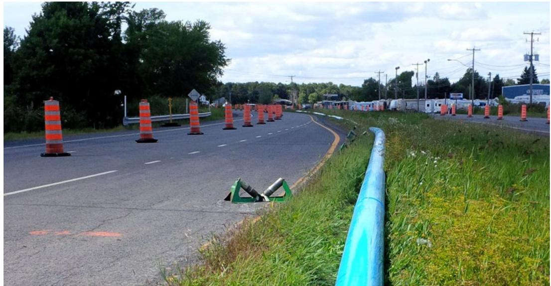
Road 104, outside the city of St-Jean-sur-Richelieu, PQ, is the first location in the province of Quebec to install large diameter (14") Bionax® pipe. But Bionax was only part of the seven kilometer story.
