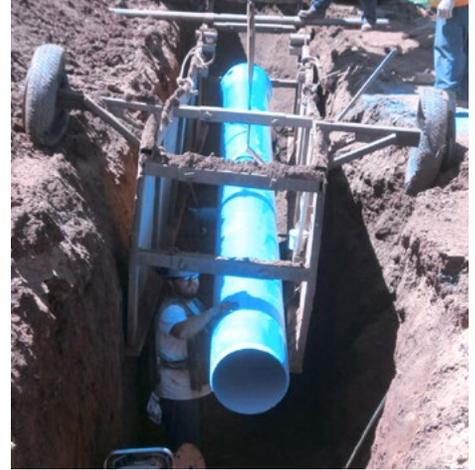
As a PVC-friendly city, Summerside, Prince Edward Island (PEI), planned to use PVC pipe as it began Phase II of its Pope Road watermain expansion project. The project required 300 meters of 400 mm (16-inch) pipe, and was taking place in an area of the city with no existing water line.
