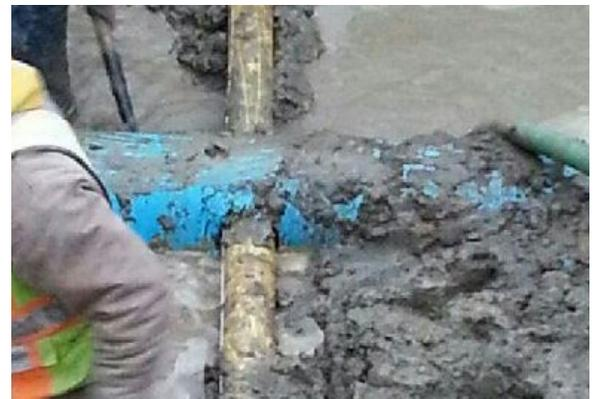
This experience is an example of how Bionax's unique material structure encourages failures to remain local and limits the size of the area to be repaired.
