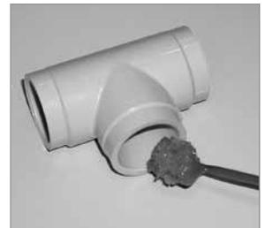
Special care shall be exercised when assembling BlazeMaster systems in extremely low temperatures (below 4°C (40°F)) or extremely high temperatures (above 38°C (100°F)). Extra set time shall be allowed in colder temperatures. When cementing pipe and fittings in extremely cold temperatures, make certain that the cement has not "gelled". Gelled cement must be discarded. In extremely hot temperatures, make sure both surfaces to be joined are still wet with cement when putting them together.
