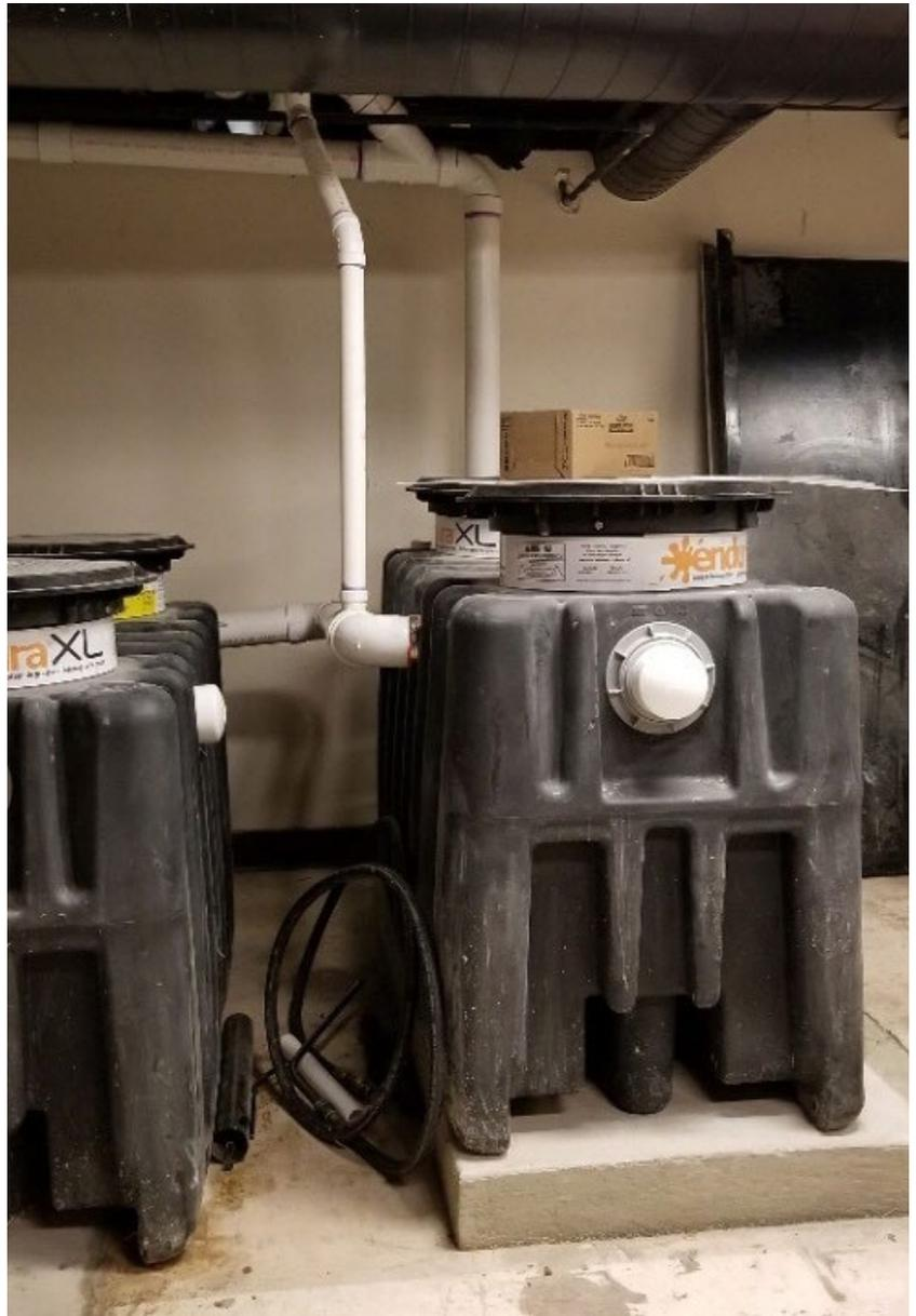
Two Endura® XL100 Grease Interceptors were installed in the basement of Half-Shell Oyster House
