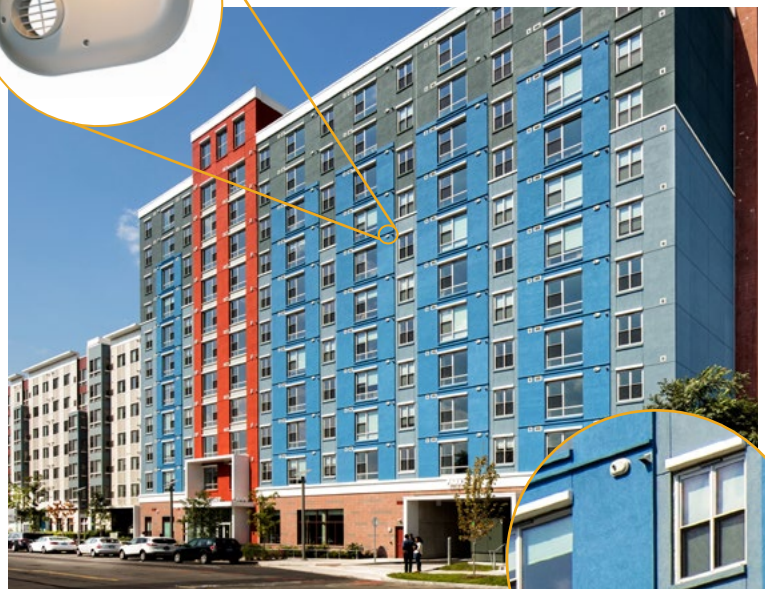
IPEX low-profile termination units with custom 3D specifications are on the building facade.
