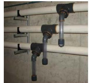
For more than 20 years, Guardian systems from IPEX have been the benchmark in double containment piping in North America. With all the corrosion resistance, performance and longevity benefits of Xirtec140 PVC, the Guardian Vinyl double containment system improves overall safety at the Lakeview WWTP, while ensuring reliable service to the surrounding community for the life of the system.
