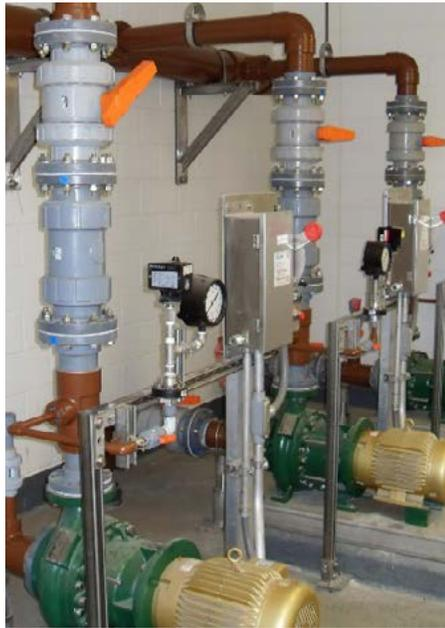
of choice. The Guardian double containment systems were comprised of approximately 2000 feet of 6-inch Xirtec®140 Schedule 80 PVC carrier inside 10-inch Xirtec140 Schedule 80 PVC containment. Another nearly 2500 feet of larger diameter 10-inch carrier inside 16-inch containment and 8-inch carrier inside 12-inch containment were also deployed.
