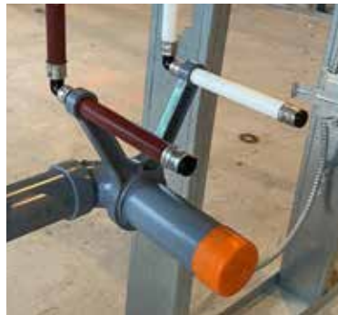
System XFR Water Line Installation
