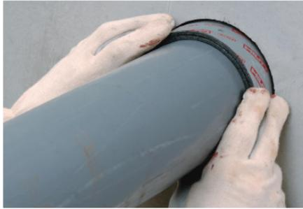
Most applications will require an F-Rating, which is typically the fire resistance rating of the assembly. However, under 3.1.9.1(2), when penetrating a firewall or under 3.2.1.2, a slab, an FT-Rating is required, which will limit the transmission of high temperatures through the assembly as well as the fire resistance rating.
