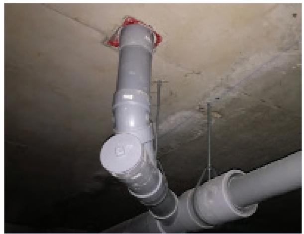
System 15 piping with a cast-in place firestop device providing a 2HR FT rating in a 3.2.1.2 parking garage slab.
