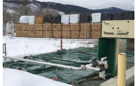
to over 5 mg/L in less than one hour. Under these aerobic conditions virtually all the existing H<sub>2</sub>S is destroyed and the high levels of dissolved oxygen prevent its re-formation.
