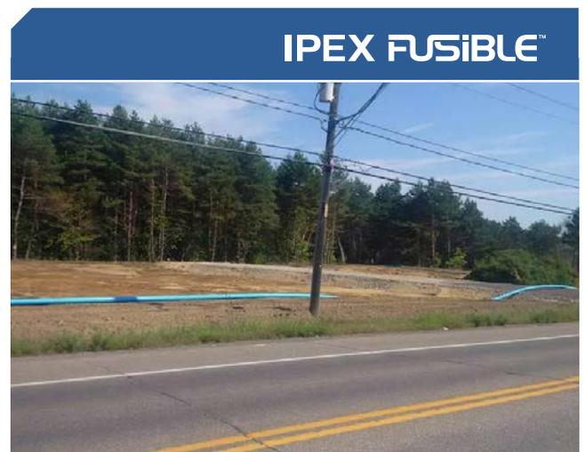
Fusible PVC DR 18 6" pipe was installed beneath the natural area.
