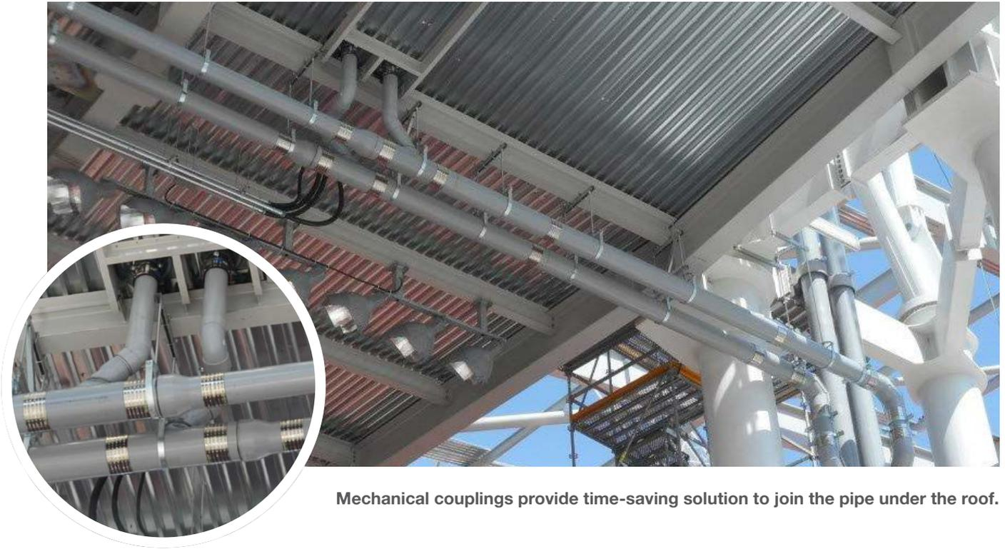
**Mechanical couplings provide time-saving solution to join the pipe under the roof.**
