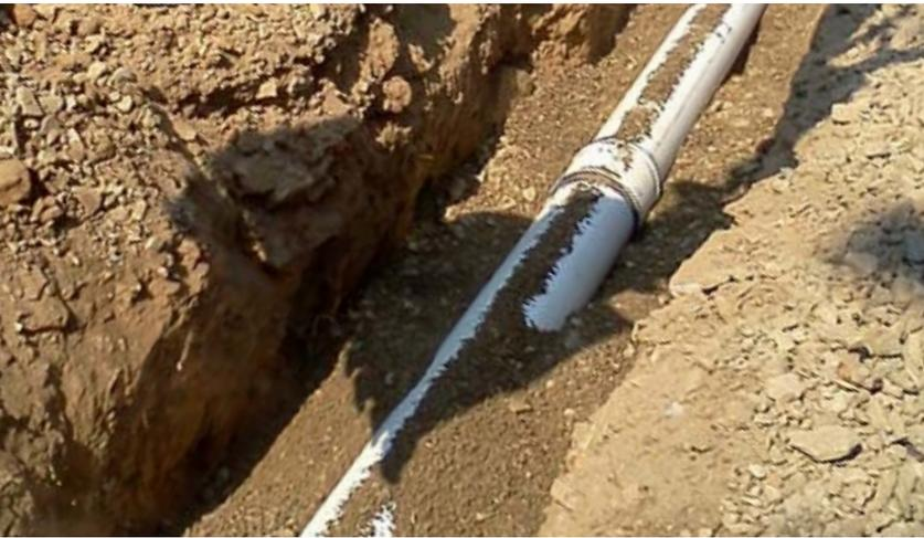
According to Lake Randall, president of Mid Penn Engineering, the IPEX Guardian Double Containment Piping System offered a far better value over other alternatives that require installing separate containment and carrier piping. “The IPEX Guardian system not only saves on installation, but it is also a higher standard for leak prevention,” he says. “PVC is resistant to chemicals, while still being able to handle the pressures of a pumping system like what was used at CAES.”
