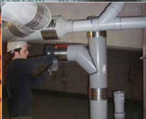
IPEX not only provides a superior alternative to cast iron, it is easy for a crew to transition their skill set from installing cast iron to PVC systems virtually overnight. With both onsite and online solvent cement training and 24/7 technical support, why go with any other DWV system?
